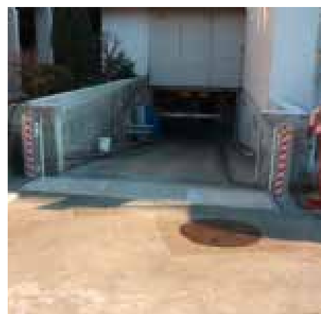
Cloison étanche rabattable, centre commercial COOP Bärenmatt, Reinach AG
