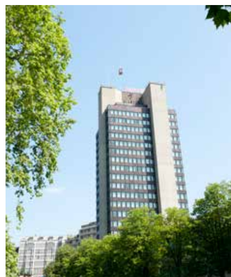
Mariott Hotel Zürich Assainissement Source: JOMOS
